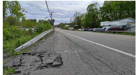
Figure 44: Severely broken pavement in shoulder on 9W northbound at Milton Road, looking south
