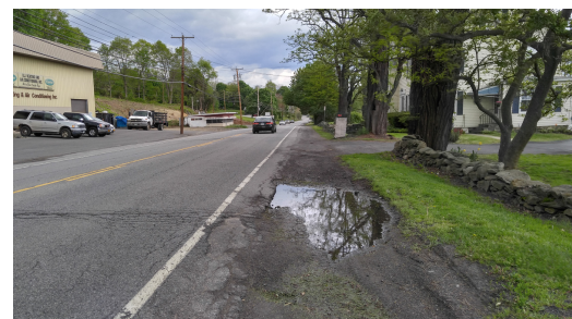
Figure 25: Unmaintained shoulder on 9W northbound between Hudson Banks and James Street, looking north
