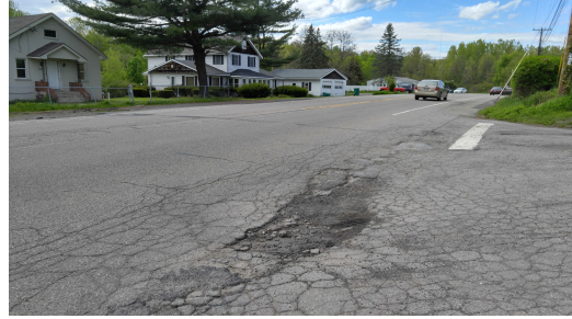
Figure 46: Moderately breaking and cracking pavement in shoulder on 9W northbound at Blue Point Road, looking north
