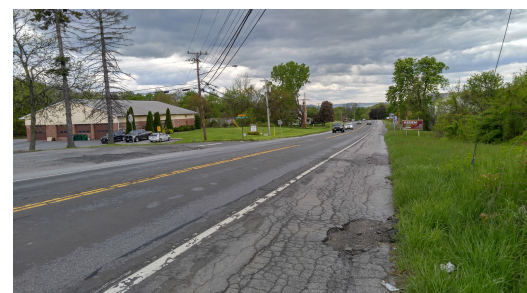
Figure 31: Some cracking and broken pavement north of Hudson Bluff Drive on 9W southbound, looking south
