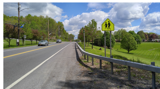
Figure 24: 8-foot shoulder in good condition along Elementary School frontage on 9W northbound, looking north
