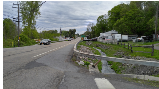
Figure 43: Shoulder in fair condition and guardrail at edge with ditch/creek below on 9W southbound at Perkinsville Road, looking south
