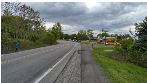
Figure 26: Shoulder in very poor condition along 9W northbound near Bixby Lane, looking north
