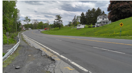
Figure 35: Narrow shoulder in poor condition with broken pavement on 9W northbound across from Ship Lantern Inn, looking south
