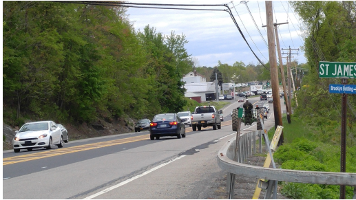
Figure 38: Slightly wider shoulder in fair condition; road narrows to one lane, shared with tractor on 9W northbound, looking north
