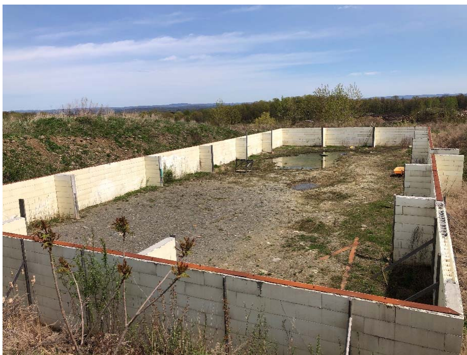
Photograph 5. Foundation frost walls at the Project Site, facing east. Photo taken on 4/29/19.
