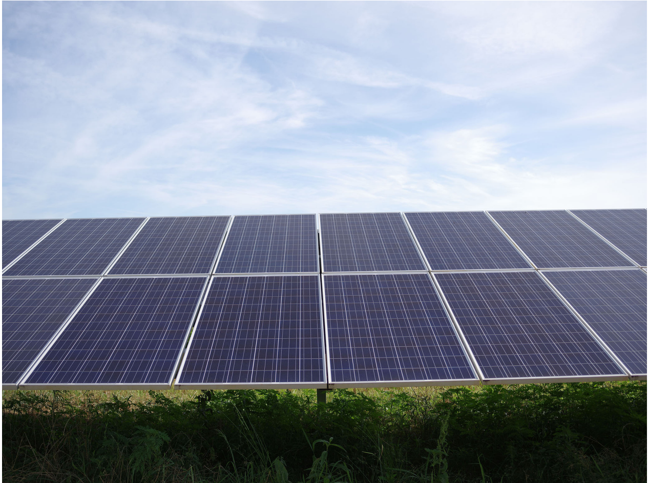
Photo 6: Ground-Mounted PV Modules 1
