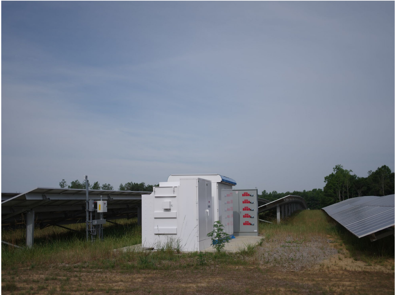
Photo 4: Central Inverter & Equipment Pad
