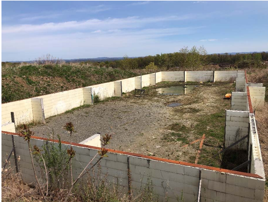
Photograph 5. Foundation frost walls at the Project Site, facing east. Photo taken on 4/29/19.
