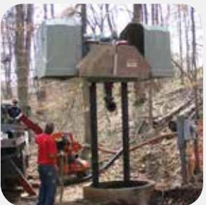
Upon delivery, simply connect suction and discharge piping and electrical connections, and secure the baseplate to the wet well. The process is typically completed within a few hours. S&L startup assistance is available.
