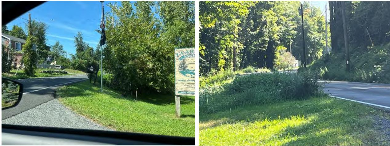
13. Similarly, the sight distance onto Ridge Road appears excellent looking to the right but limited to less than 200 feet due to vegetation immediately north of the driveway (image, below, left). A southbound driver may only see a car's front bumper pulling out due to the vegetation (image below, right). Although the applicant recommends an intersection warning sign, additional effort should be provided to mitigate this condition.
