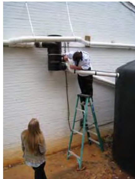
Figure 2.3.2 Inspecting the Conveyance System and a Vortex-style Filter
