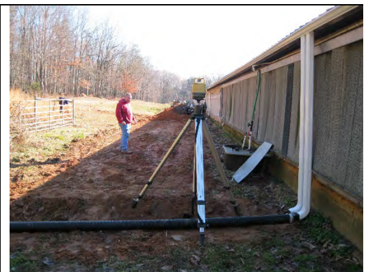
Source: Rainwater Management Solutions 1 Example of enhancing the gutter and piping system leading to a rainwater harvesting system
