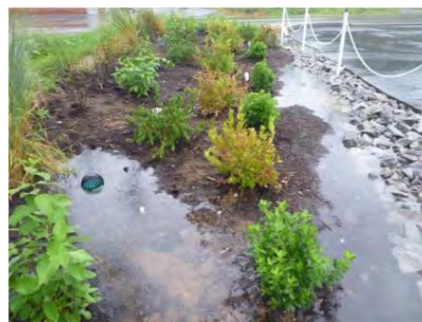
Water is preferentially ponding only at one end of the bioretention because the surface is not flat.
