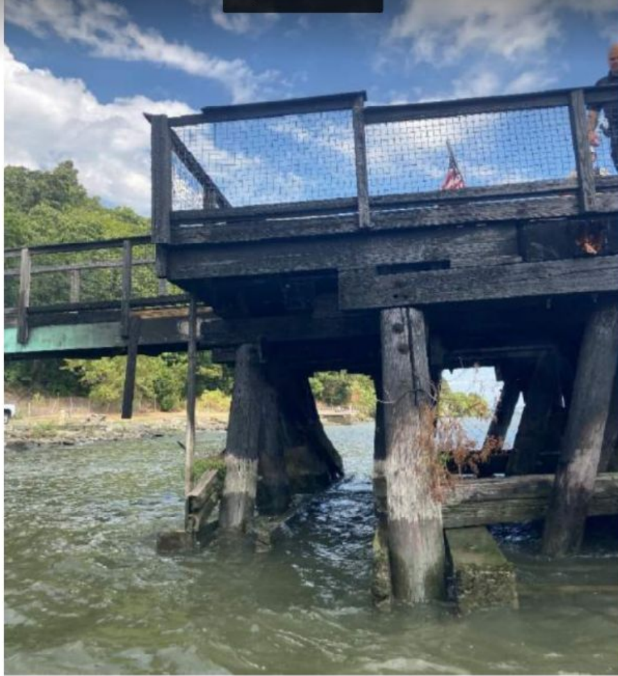
Photo 5: \frac{3}{4} " Split In Top 4' of Pile 2A Batter South, Looking North
