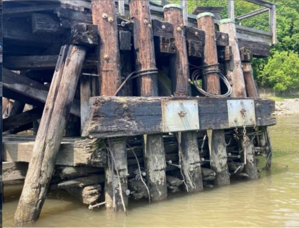
Photo 9: 1" Split in Fender B-Batter South, Looking Northwest
